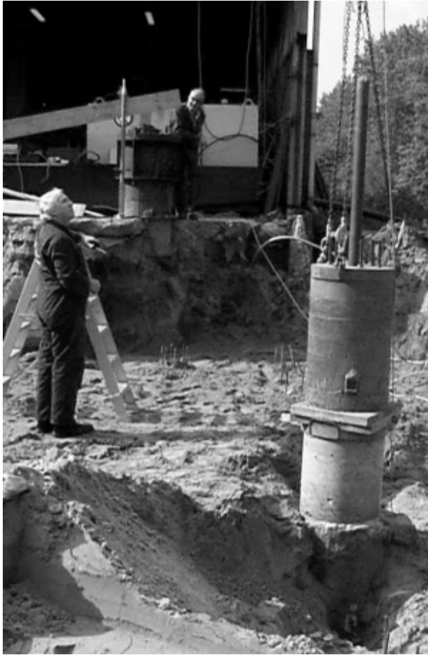
Fig. 2. Dynamic load test on a cast in situ pile.
