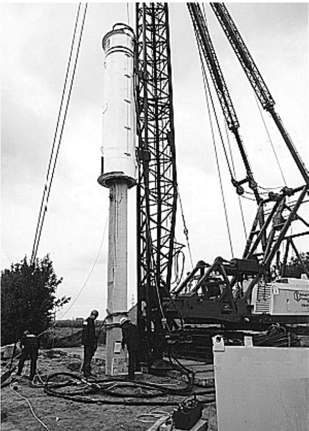
Fig 9. Dynamic load test on a pre-cast pile
