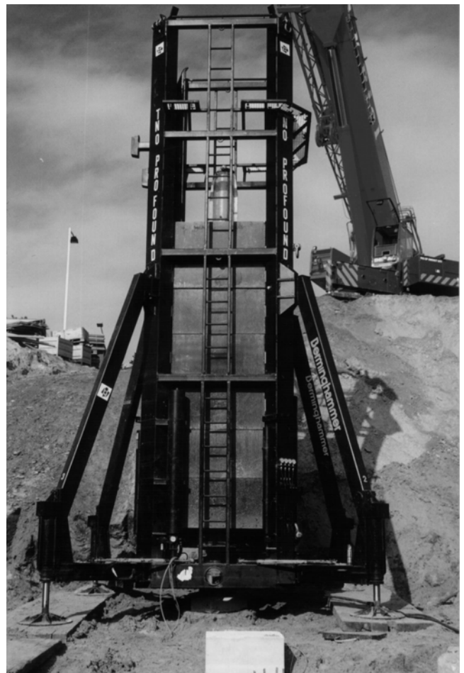
Fig. 1 statnamic test on a cast in situ pile
