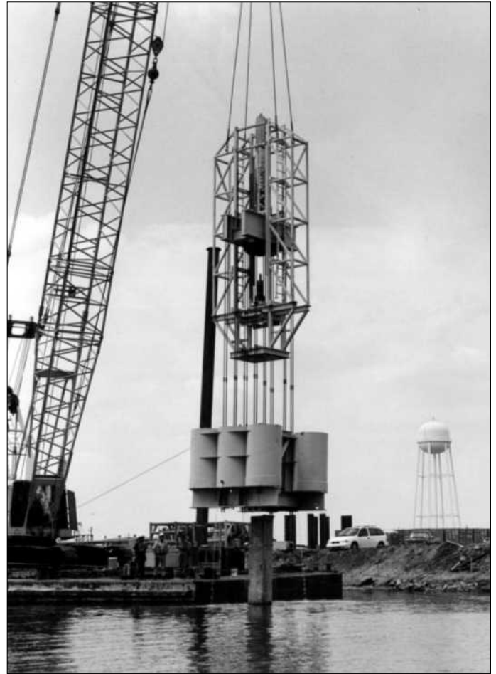
Figure 7 Statnamic equipment being placed on a test pile
