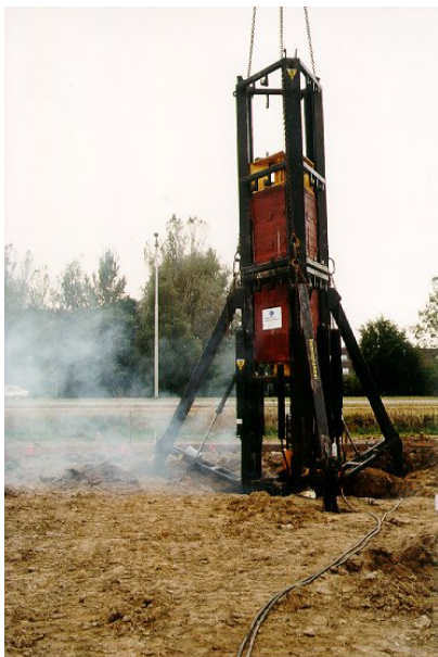
Fig. 1 statnamic test on a cast in situ pile
