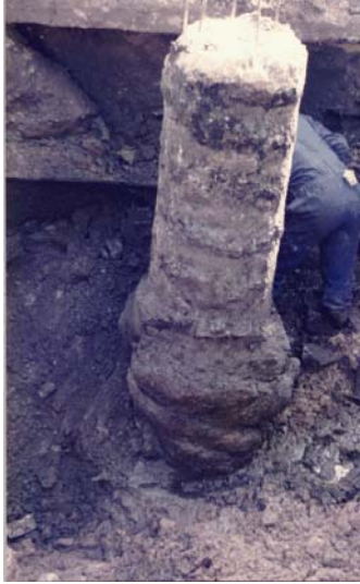
Fig 8. Cast in situ pile with bulb
