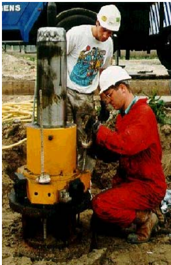
Fig. 3. Statnamic piston with built in load cell placed on a cast in situ pile
