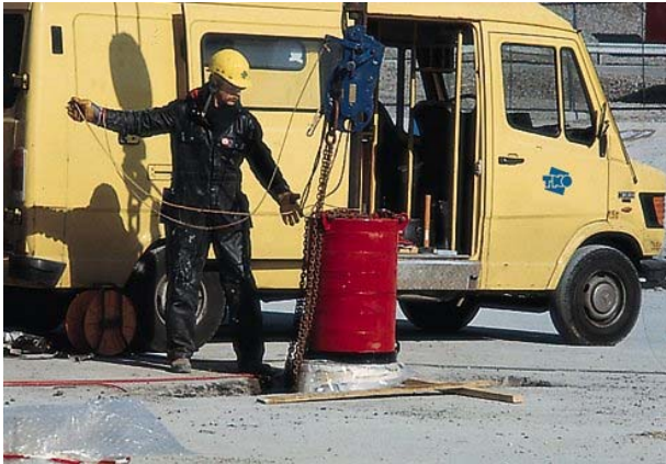
Fig. 2. Dynamic load test on cast in situ pile
