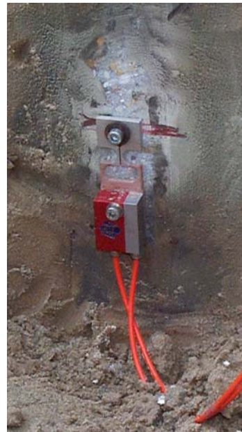
Fig. 4. Strain transducer mounted on the shaft of a cast in situ pile
